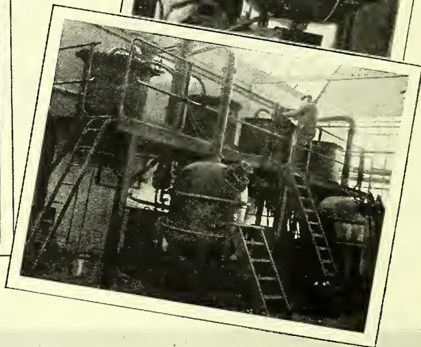
Extractors and Recovery Stills
